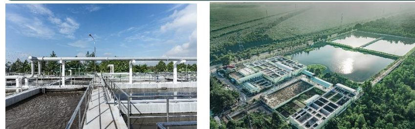
IDICO's IPs are uniformly developed with treatment facilities to recycle wastewater and maximize run-off capture
