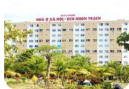
Workforce housing project in Nhon Trach 1
