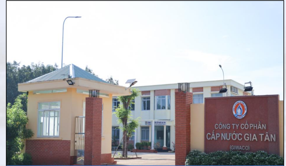
GIA TAN WATER PLANT (DONG NAI)
