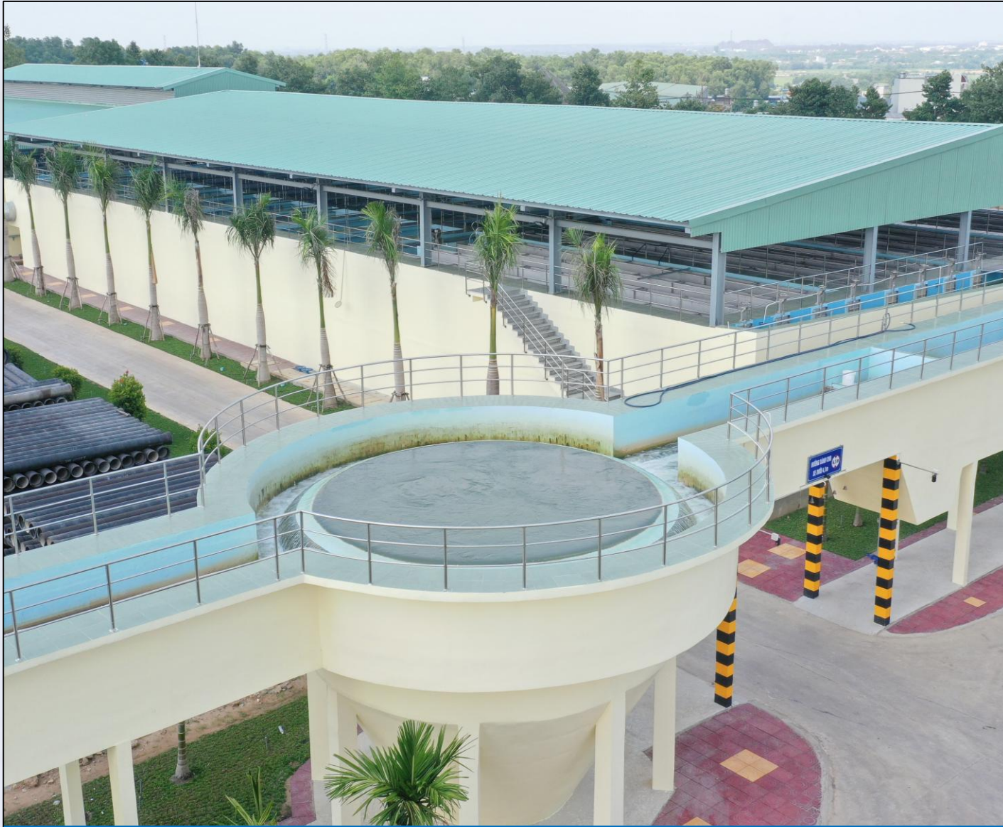
DI AN WATER SUPPLY BRANCH WITH A CAPACITY OF 300,000 M3/DAY
