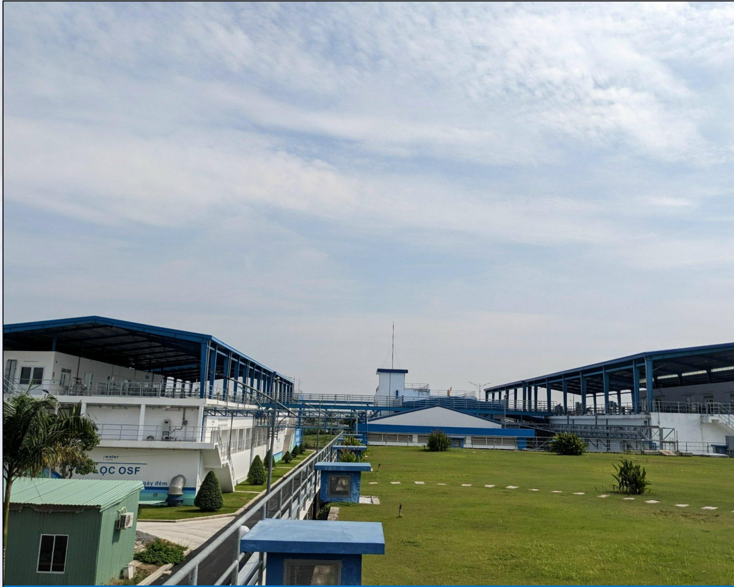
NHI THANH WATER PLANT (LONG AN)
