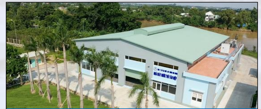
TAN HIEP WATER PLANT
