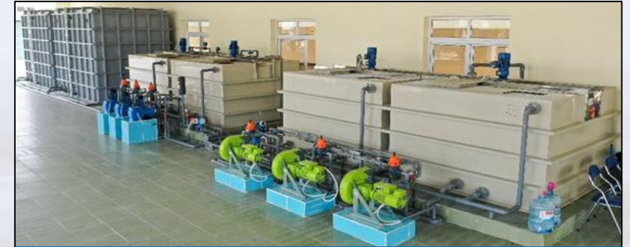
CHEMICAL HOUSE (PAC AND LIME) – FULL AUTOMATION
