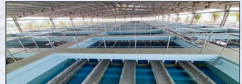
SEDIMENTATION TANK
